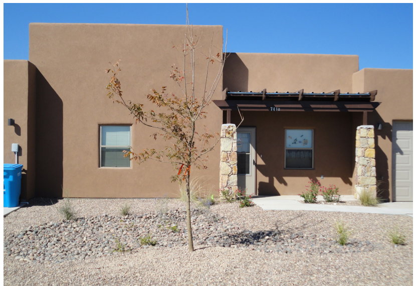
Photo Courtesy: Bryan Schuler, Travois The Ysleta del Sur Pueblo tribe used LIHTCs to develop 30 duplexes in Socorro, Texas.
