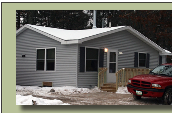
Pictured: College of Menominee Nation students helped renovate this home to make it handicap accessible, through a partnership with the Menominee Tribal Housing Department.
