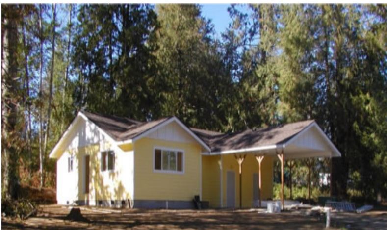
A home built with low income housing tax credits on the Lummi Reservation in Washington state.
