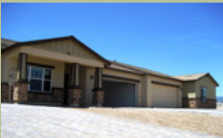
Top: Enclosed two car garages and covered porches are definitely welcomed by tenants in the hot Arizona climate.
