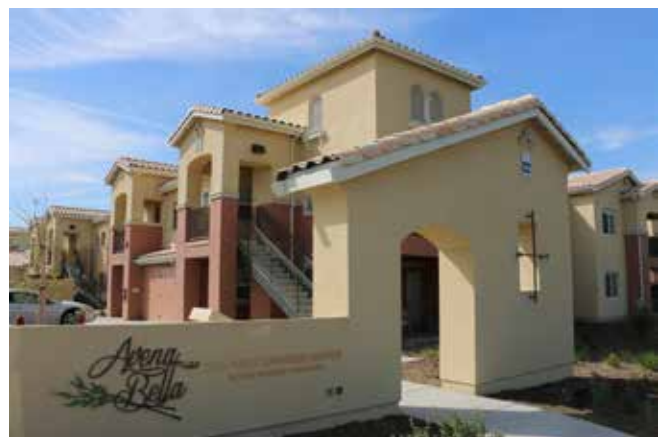
Photo: Courtesy of EAH Housing Avena Bella
